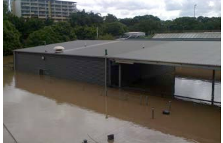
o2a: The University of Queensland Boating and Diving shed during January 2011 flood event.
