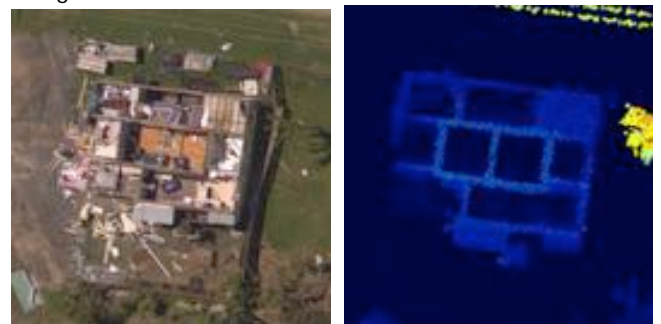
Figure 2. Damage to building in Yeppoon.
